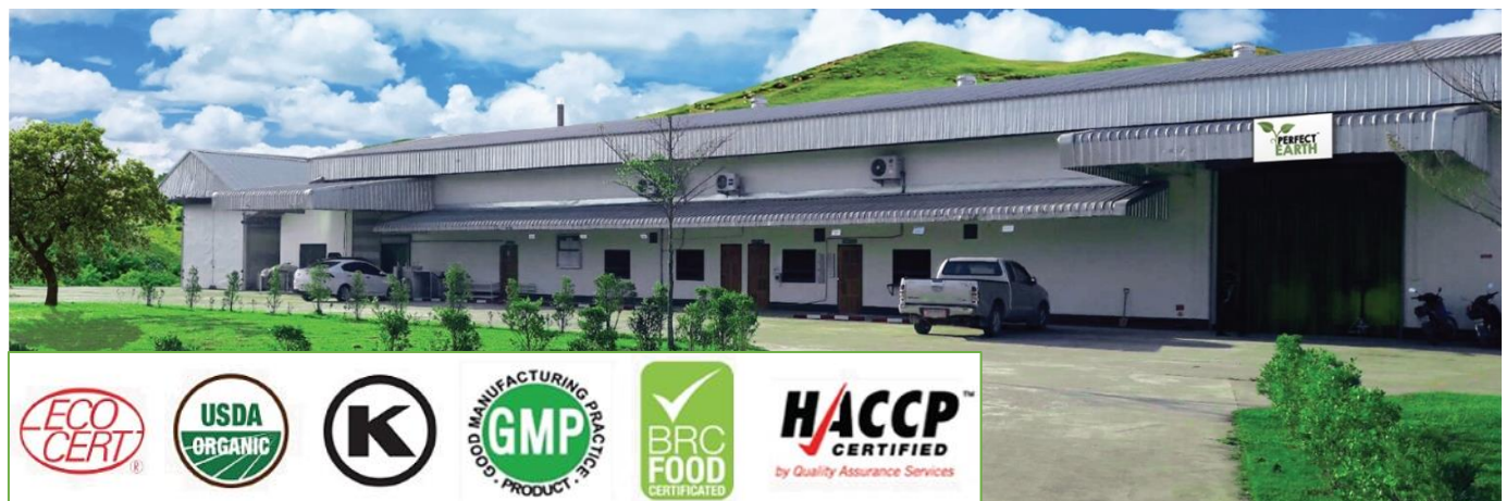
Figure 4: Chacha Chiang Rai existing production plant and global certifications
