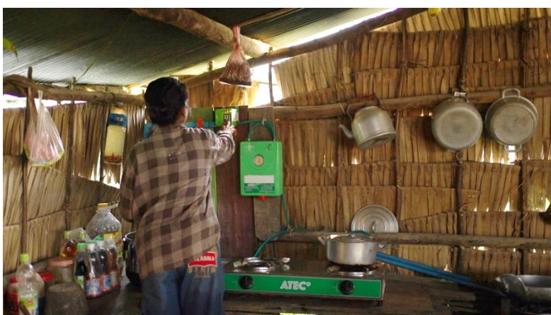
Figure 2 A biogas stove linked to a PAYGO panel
